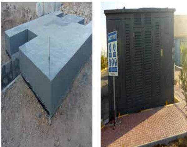
CONCRETE FOUNDATION FOR PACKAGE SUBSTATION AND RELATED CIVIL WORKS FOR ELECTRICAL TIE-IN FOR PETROTEC
