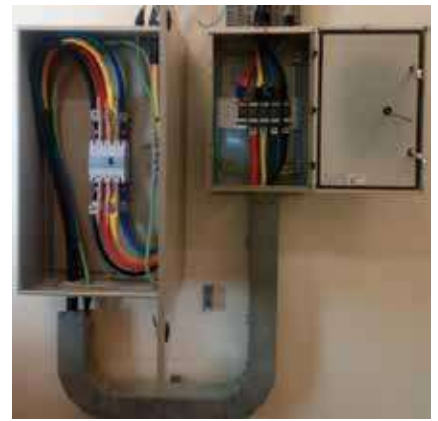
DB INSTALLATION & TERMINATION
