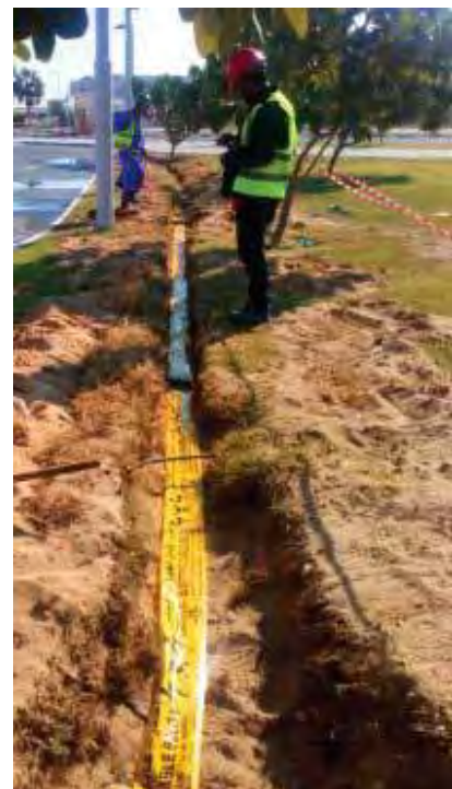
EXCAVATION FOR CABLING
