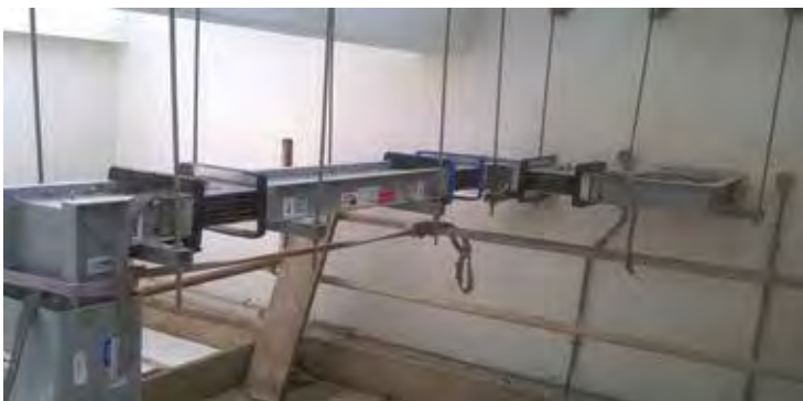
BUS BAR INSTALLATION IN SUBSTATIONS
