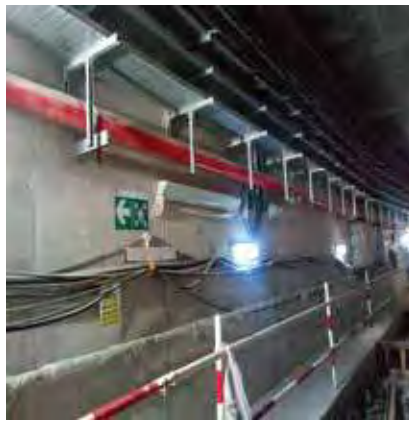
CABLE TRAY INSTALLATION
