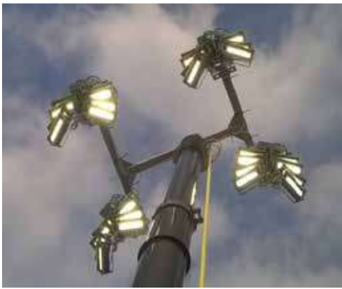
HH SHEIK JASSIM PALACE LIGHT INSTALLATION
